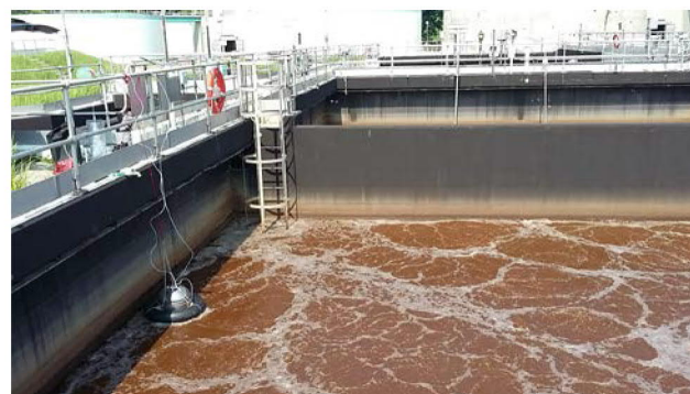
S4 - Aeration Tank Surface
