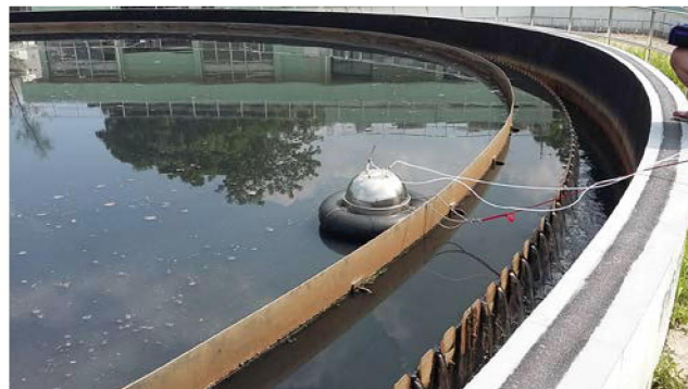
S3 - Primary Sedimentation Tank Surface
