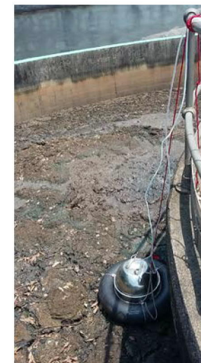
S8 - Sludge Holding Tank
