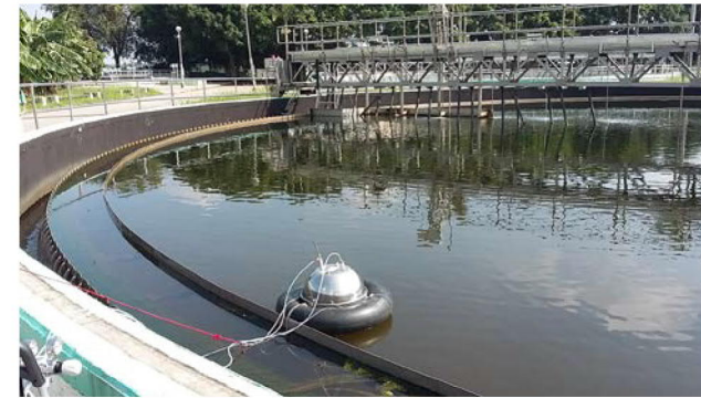
S5A - Final Sedimentation Tank
