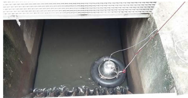
S2 - Screening Skips at Inlet Works
