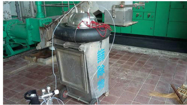
S11 - Screening Press House for Coarse Screens
