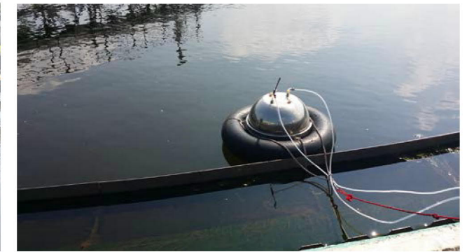
S5B - Final Sedimentation Tank
